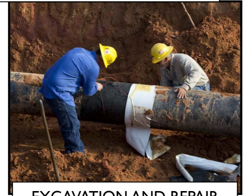
EXCAVATION AND REPAIR
